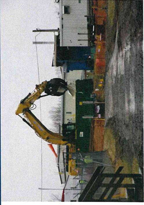
Roof being removed from VIT Hill restrooms
