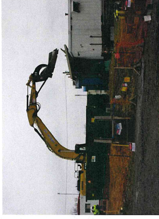
Roof being removed from VIT Hill restrooms
