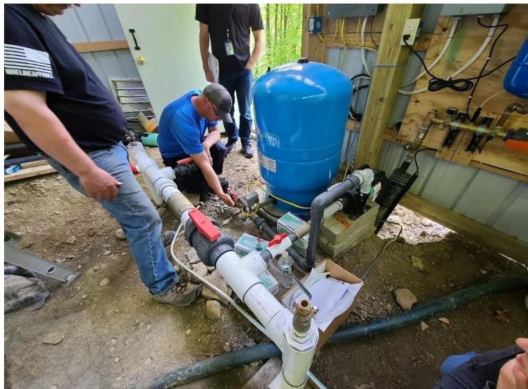
Photo showing a unique constant pressure manifold system at the reservoir site of a seasonal campground.
