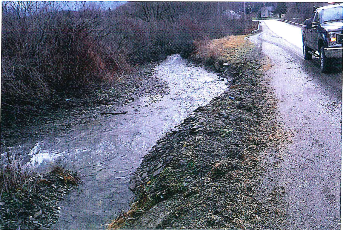
REACH 1 - LOOKING DOWNSTREAM.
