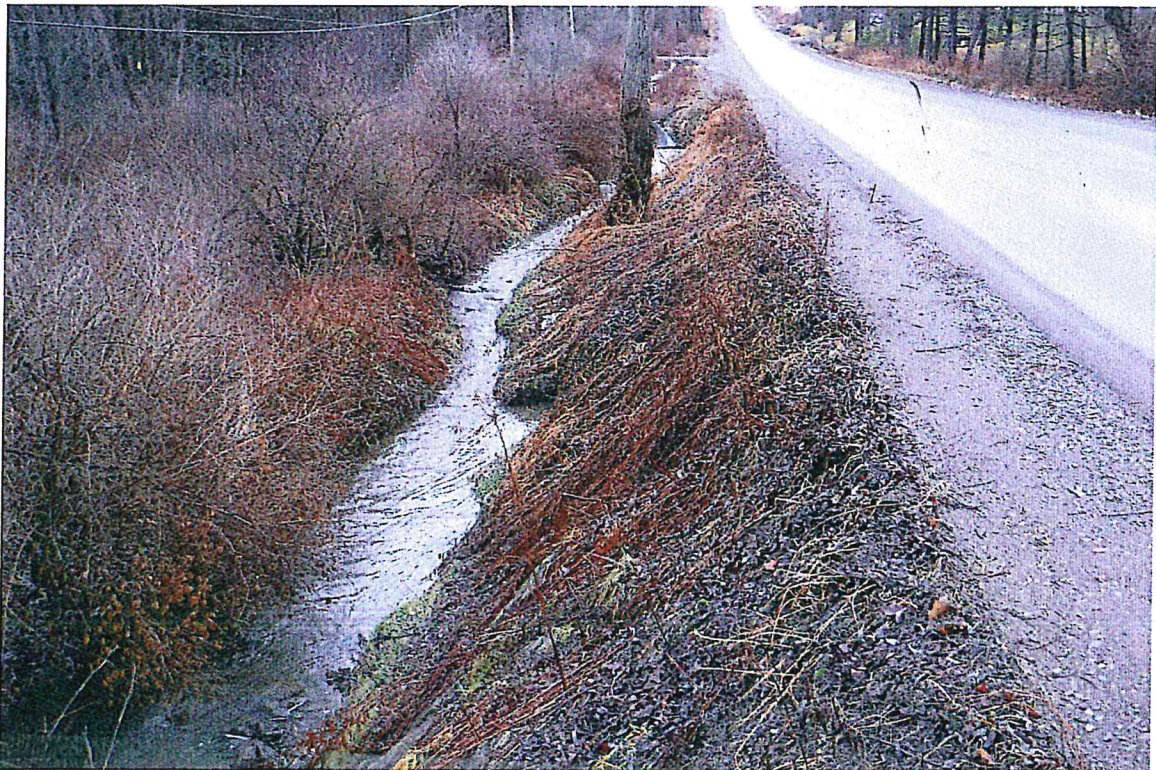
Co Rd #47 LOOKING DOWNSTREAM
