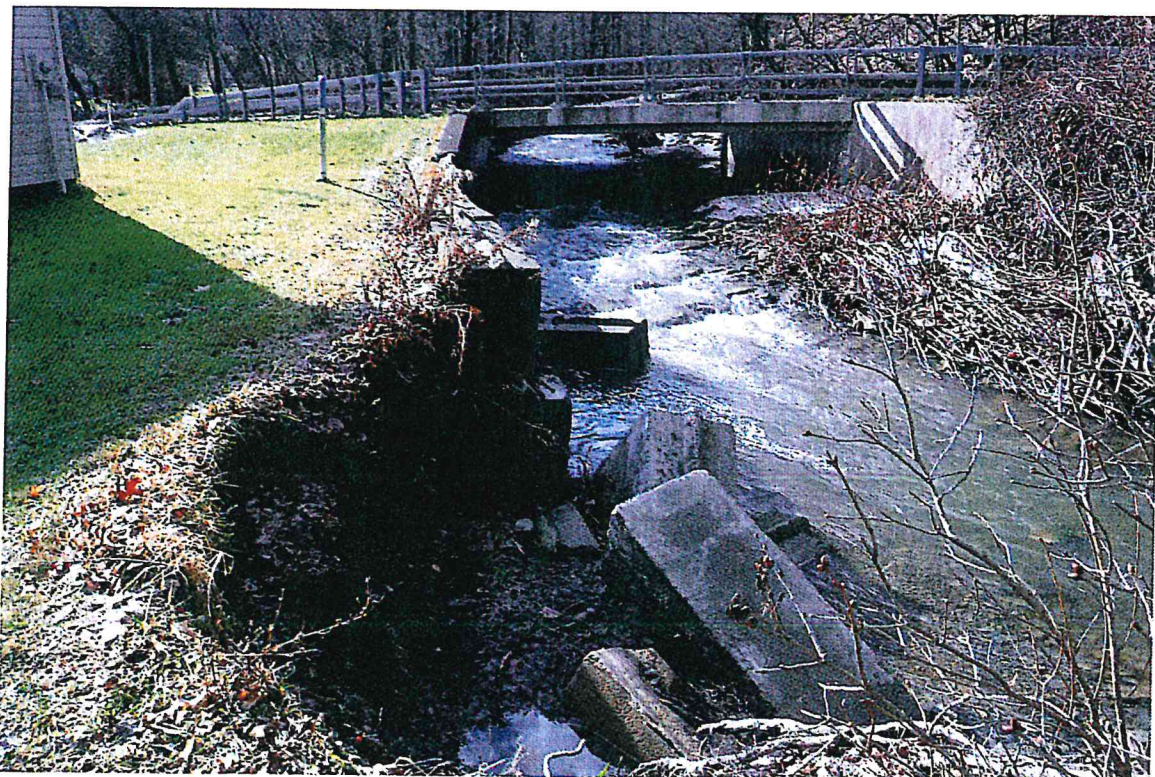
LOOKING UPSTREAM AT THE BRIDGE
