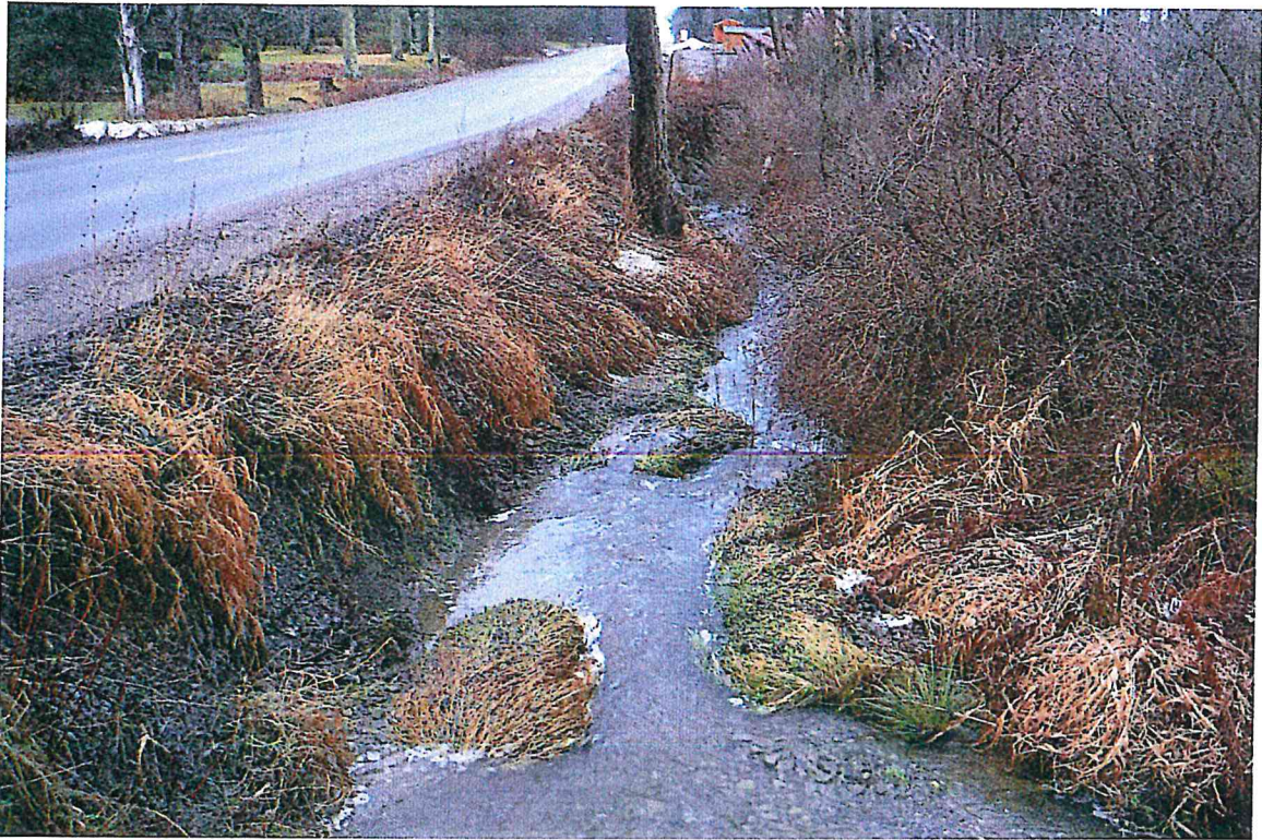
Co Rd #47 LOOKING UPSTREAM
