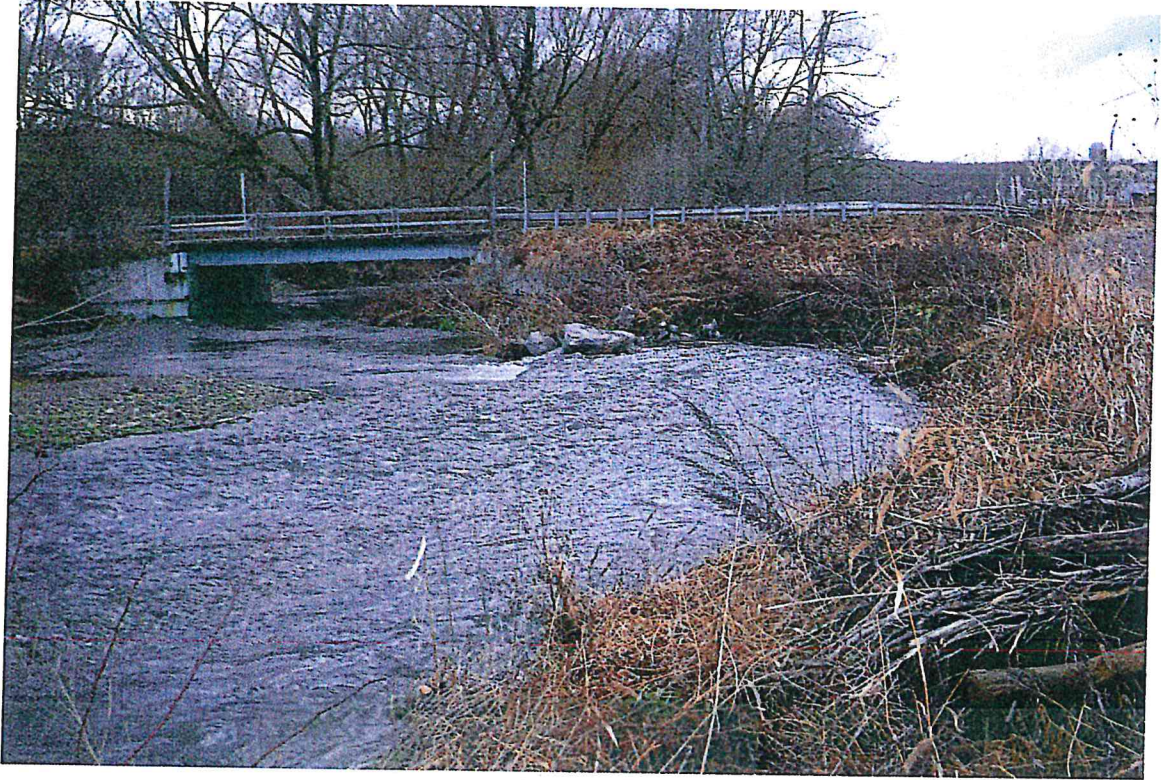
LOOKING UPSTREAM AT TOWN HILL ROAD
