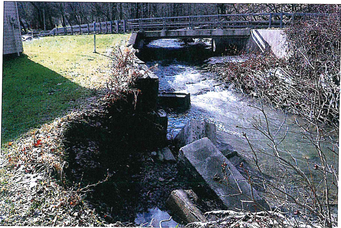
LOOKING UPSTREAM AT THE BRIDGE
