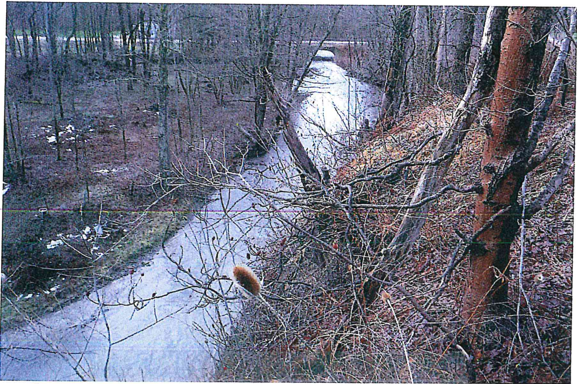
CR 32 LOOKING DOWNSTREAM
