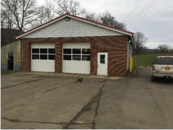
Sewer Treatment Plant Garage
